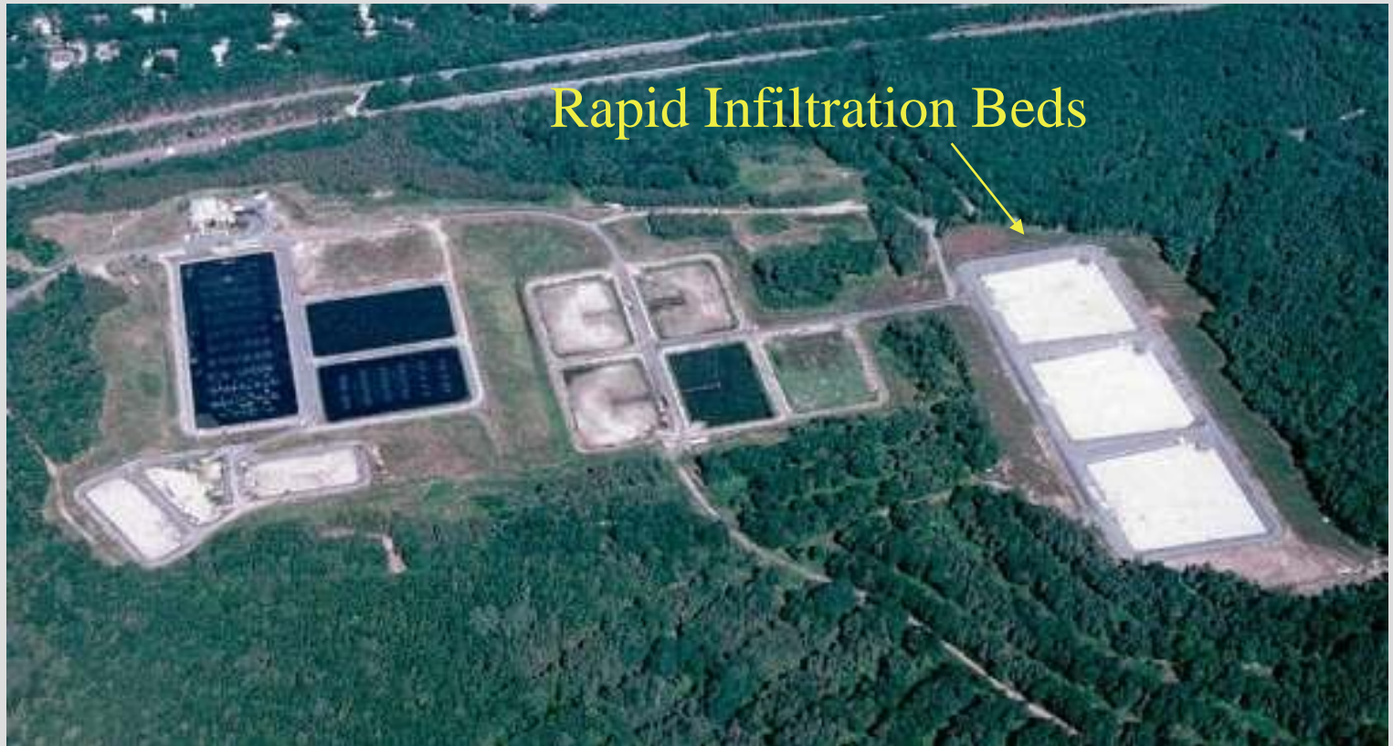
Falmouth, MA – 0.8 mgd facility
